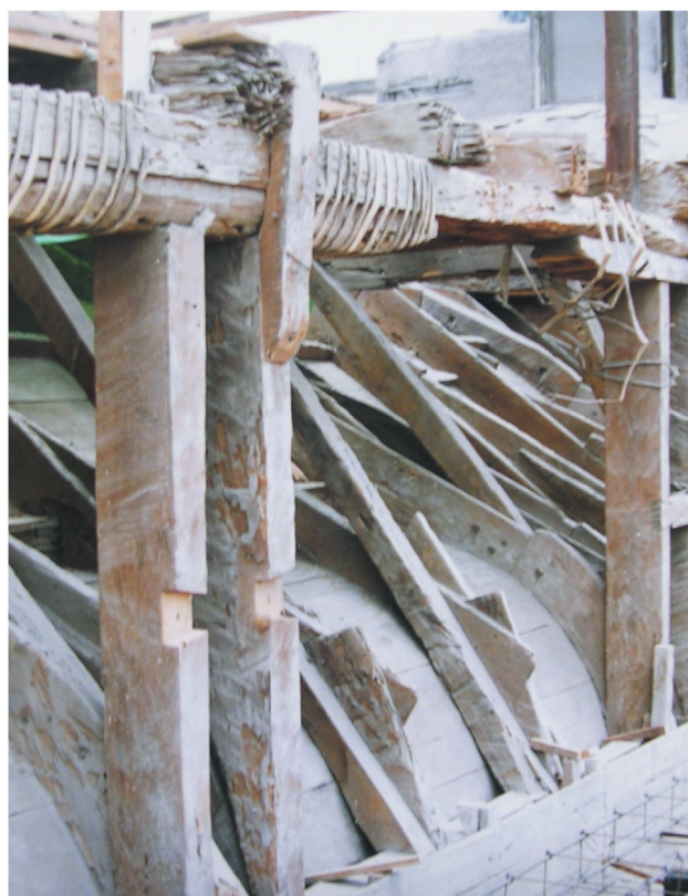
Figure 13. Wooden vault according to the lintel system in the Virgin of Loreto’s chapel in Lima, Peru.
