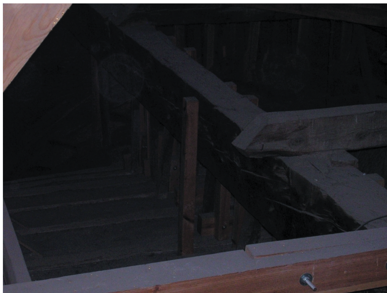
Figure 10. Planked timber vault in Saint Anton church in Madrid built with Spanish techniques.
