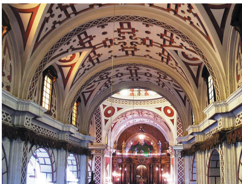
Figure 11. Planked timber vault in Saint Francis church in Lima, Peru.
