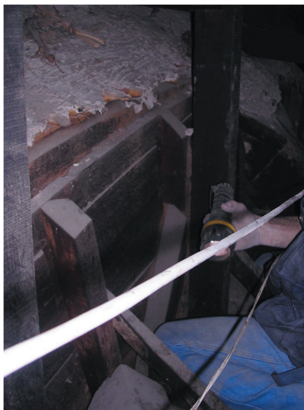
Figure 12. Planked timber vault in the Lima cathedral, Peru.
